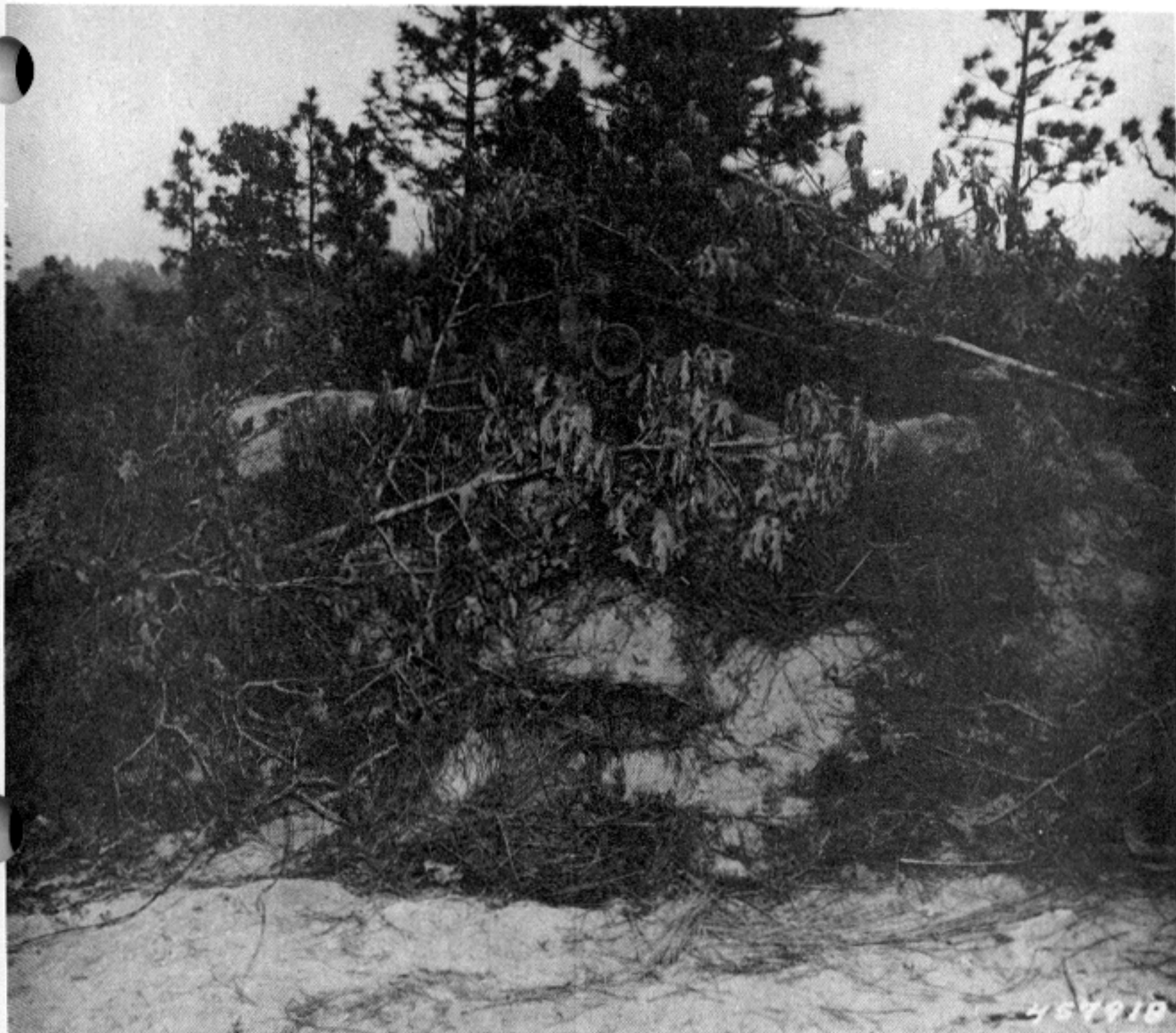
Figure 28. A roadside foxhole with a 3.5 rocket launcher. (Back blast from such recoilless weapons as the rocket launcher must be considered when locating and constructing emplacement.)
